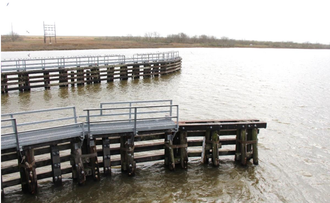
Condition Photo 7: South timber fender system with catwalks.
