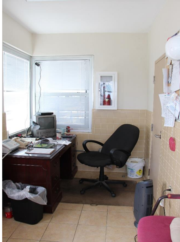
Condition Photo 11: Tile, paint, and windows in the operator's house from 2011 rehabilitation.
