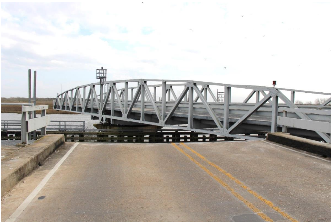
Condition Photo 16: Swing pony truss opening.
