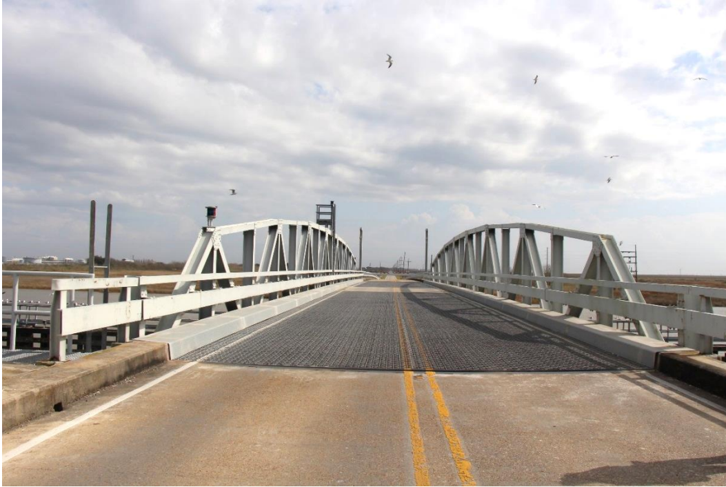
Condition Photo 15: Swing pony truss looking east.
