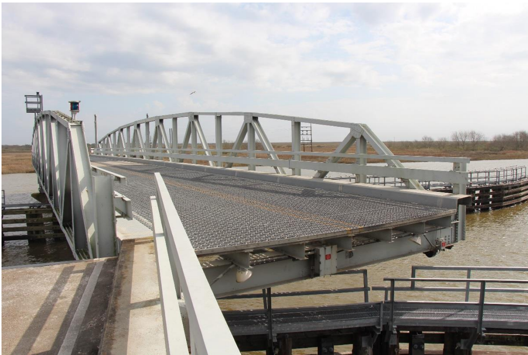
Historic Fabric Photo 4: Truss floor system.
