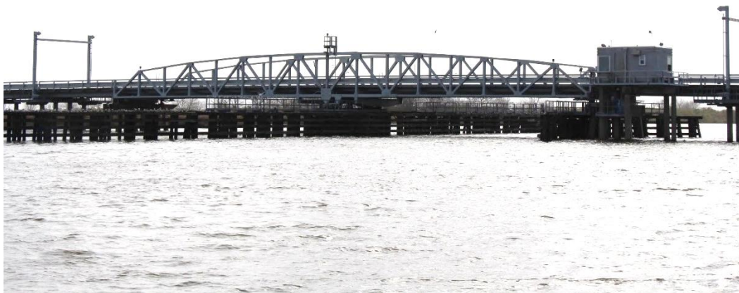
Character-defining Feature Photo 1: Design and construction of the Warren pony truss swing main span.
