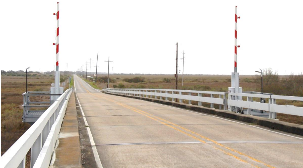
Condition Photo 12: East approach spans looking east.
