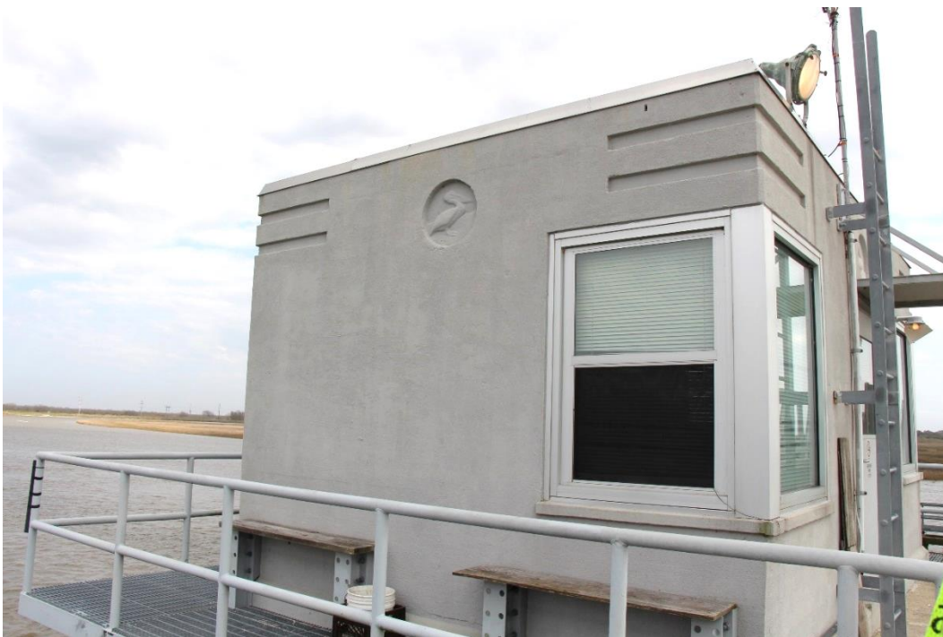
Condition Photo 8: Operator's house exterior, rehabilitated in 2011.
