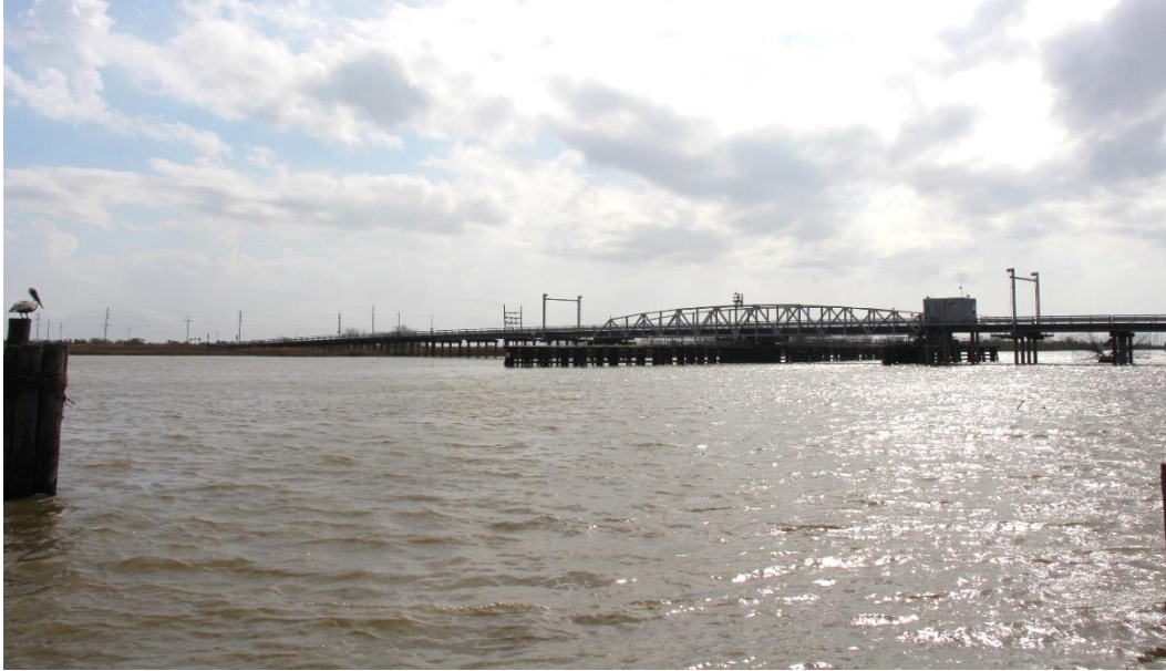
Condition Photo 19: Overall view of bridge looking south.
